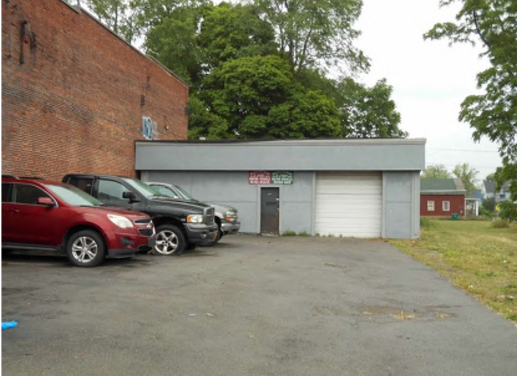
Photo 23 – 908 Genesee Street (3.1.50) - This site is currently vacant, but was previously operated as an electric motors and DLRS repair shop. The site consists of one single-story building and associated parking lot.
