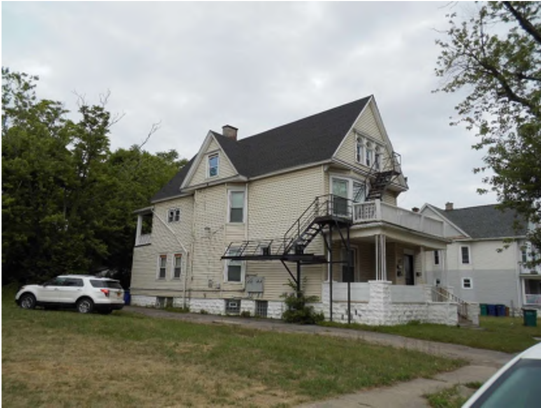
Photo 1 – 545 East Utica Street (3.1.4) - This site is currently a residential property and consists of one building and associated yard.
