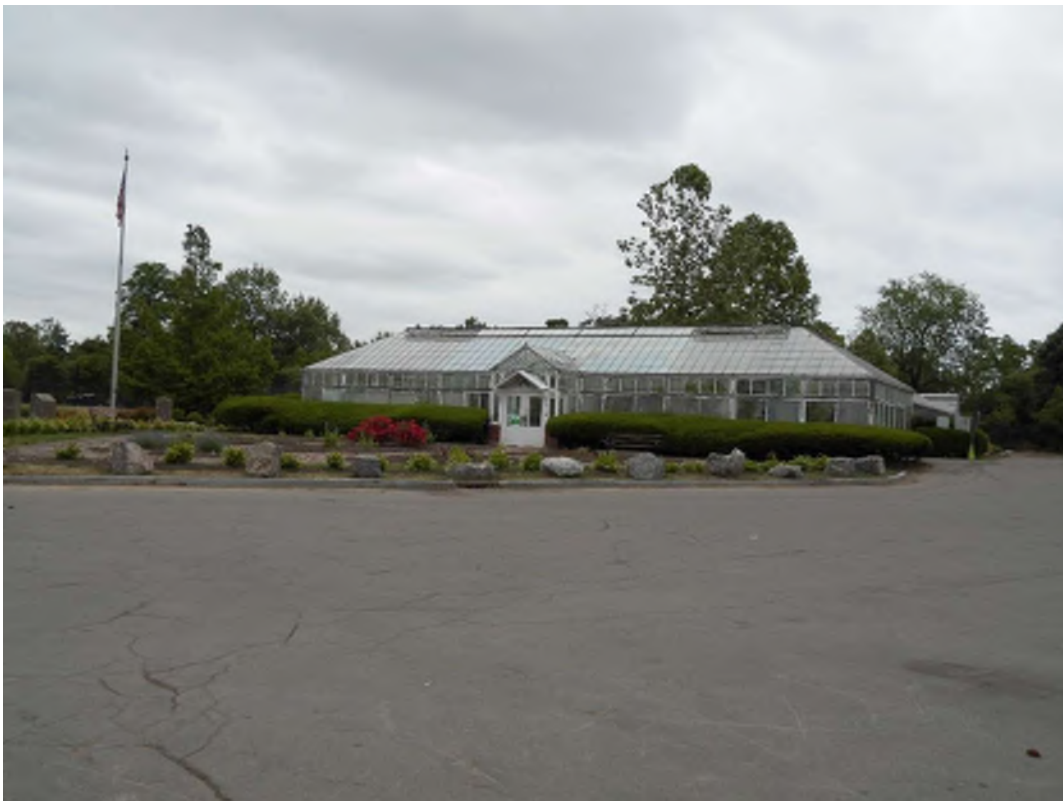
Photo 4 – MLK Greenhouse Humboldt Parkway (3.1.8) - This site is currently a greenhouse located within Martin Luther King Park and consists of one building and the surrounding yard.
