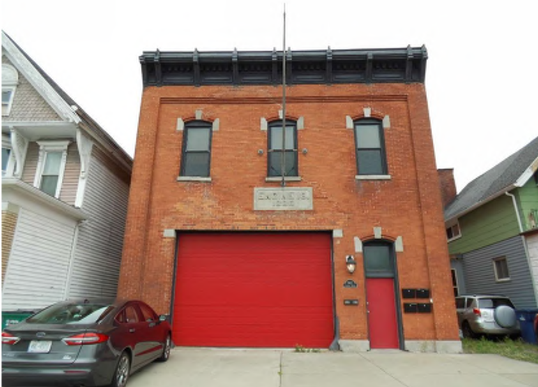
Photo 28 – 1032 Fillmore Avenue (3.2.7) - This site is currently operated as the Engine 18 Fire Station. The site consists of one building and the associated parking area.
