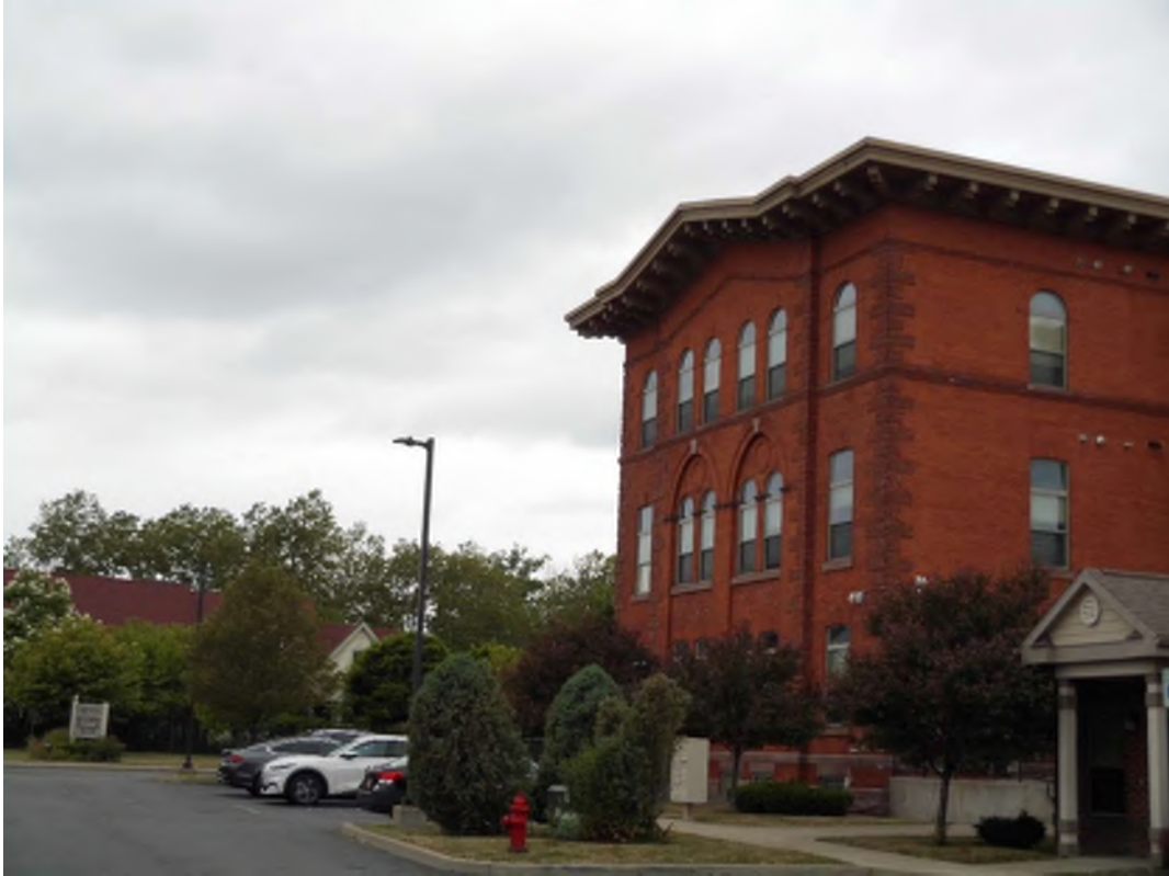
Photo 9 – 564 Dodge Street (3.1.18) - This site is currently operated by St Martin Village as a Seminary. The site consists of 11 buildings of all different shapes and sizes and associated lawns and parking lots.
