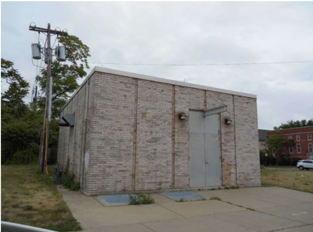
Photo 8 – 759 Humboldt Parkway (3.1.17) - This site is currently a state owned pumphouse used to prevent flooding on Kensington Expressway and consists of one building and the surrounding yard.
